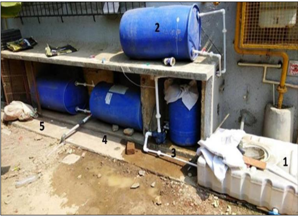
Fig 1 Constructed greywater treatment system at IWSA (1) Greywater collection tank (White), (2) Aeration tank (up), (3) Filtration tank, (4-5) Disinfection and Storage tanks for treated water
